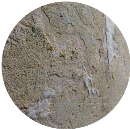
Spalling and salt efflorescences; high salt pressure
