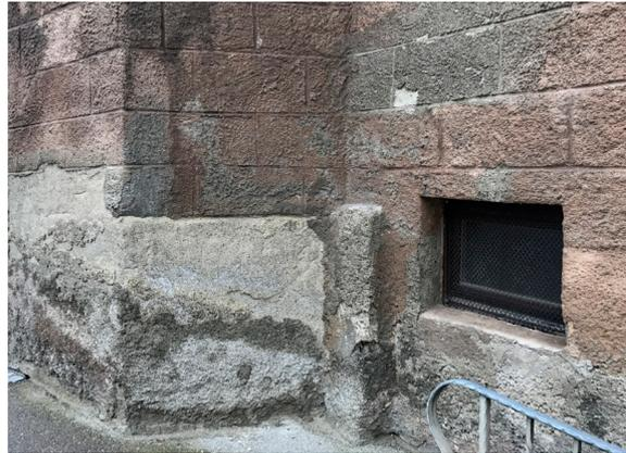
Damage patterns such as salt efflorescences and damp stains
